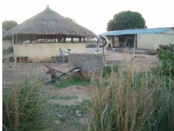
The pump, tank and main flat hose
