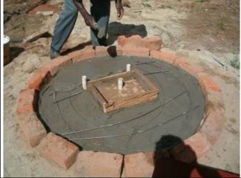
Some reinforcement bars 6 mm plus wire shopuld be placed. Not yet completed at the picture.
