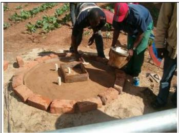
The mould is made, and tubes should be properly positioned.
