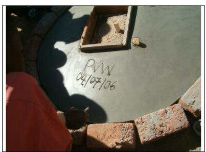
**Important:** The finished well cover should be left unused for about minimally one week for the cement to cure. The cover should be kept wet, continuously!
