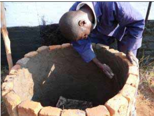
Make bricks wet, before applying cement
