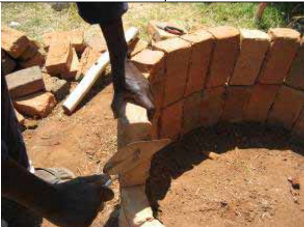
Place 2 nd round of bricks, Scrape of a little from edge to safe on cement
