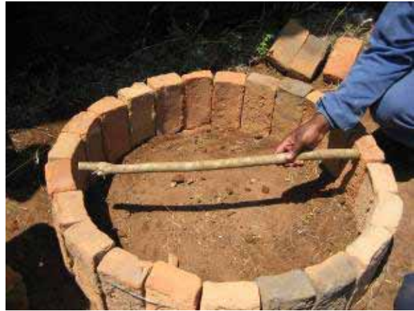
Measure with a stick to make sure the circle is round. Mount 2 more wires
