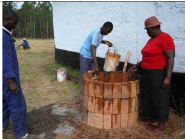
Measure with a stick to make sure the circle is round. Mount 2 more wires
