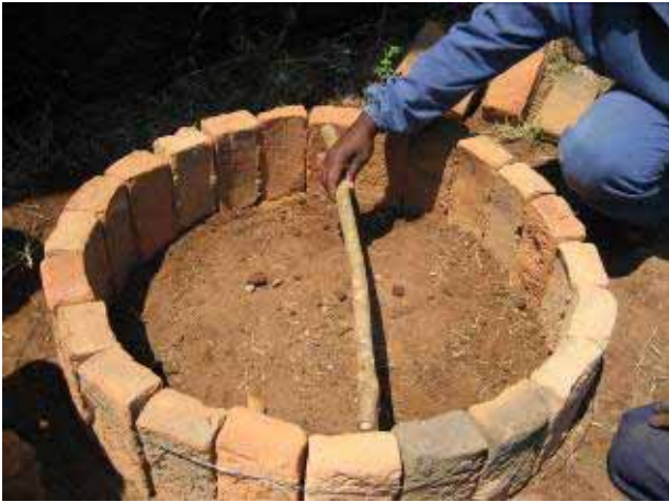
Prepare surface, Horizontal Draw a circle. Place bricks, Mount 1 st wire 3 cm from top
