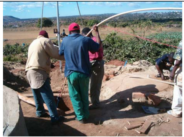
Installing the pump for the wind pump in Chimoio
