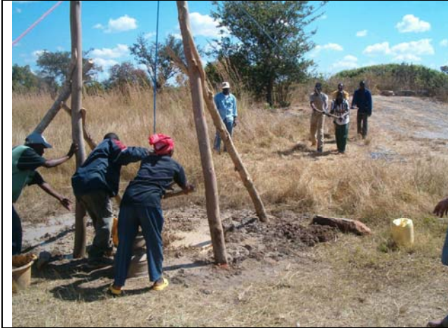
The Tanzanian drilling team demonstrating the rota sludge method.
