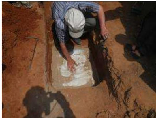
***Mount 4 ropes in the corner of the cloth filter to lift it when it needs cleaning***
