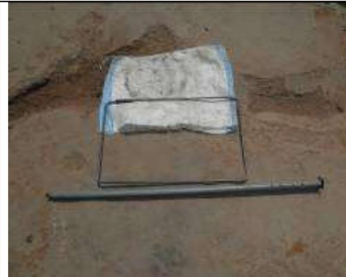
***On top of the sand a cloth filter is placed made of a maize bag and a ring of 12 mm round steel bar***
