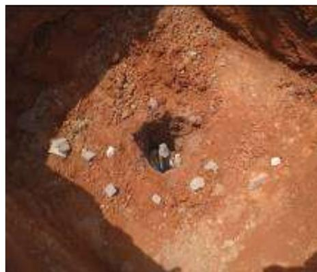
*Fill up the 2 inch hole with gravel or course sand till 2 meters from the top and place the PVC filter*
