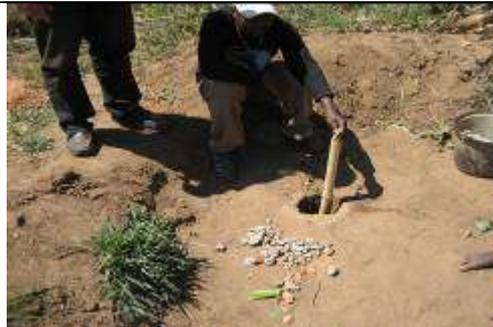
*The assembled parts are placed in the hole, than filled up with gravel, at the top sealed with clay*
