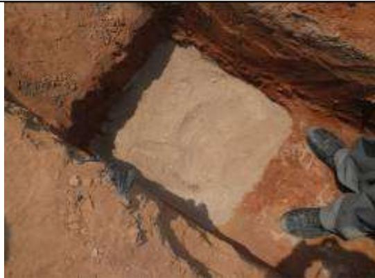
***Then the filter pipe is covered with fine sand***
