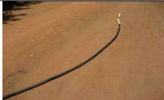
*The pressure pipe is made of a PVC pipe or in this case a black poly pipe*
