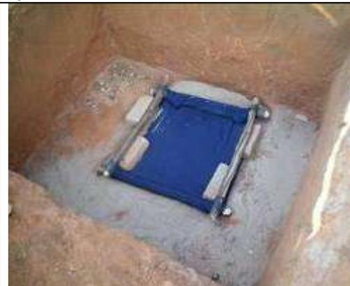
***In case the cloth filter is made of Wood, put bricks on top to avoid that the cloth filter starts floating.***
