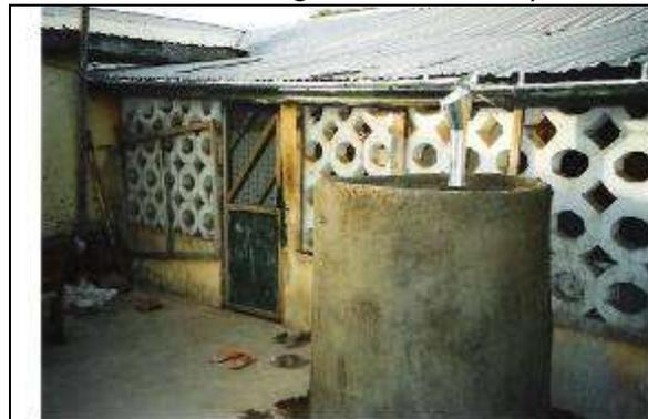
**Example in Ghana. Here a low cost Ghana gutter system is installed; water enters in a wire cement storage tank of 1 m<sup>3</sup>. The lower part of the tank is used for storage**
