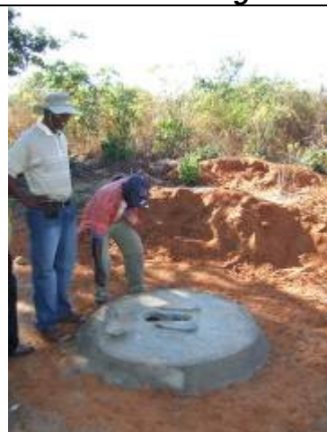
The two latrines being installed
