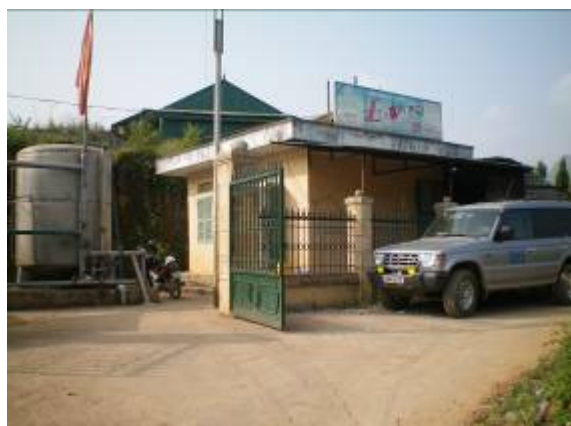
Workshop of the Lai Chau water company
