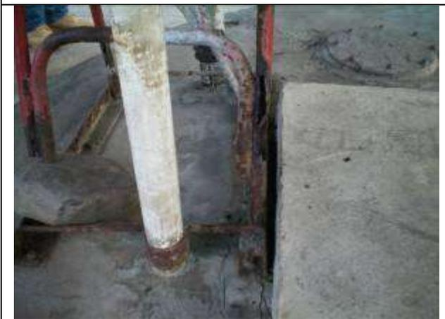
*There is much difference in quality. Pumps with black steel pipes are corroded within 10 years. Models with galvanised pipes last 20 years or more*
