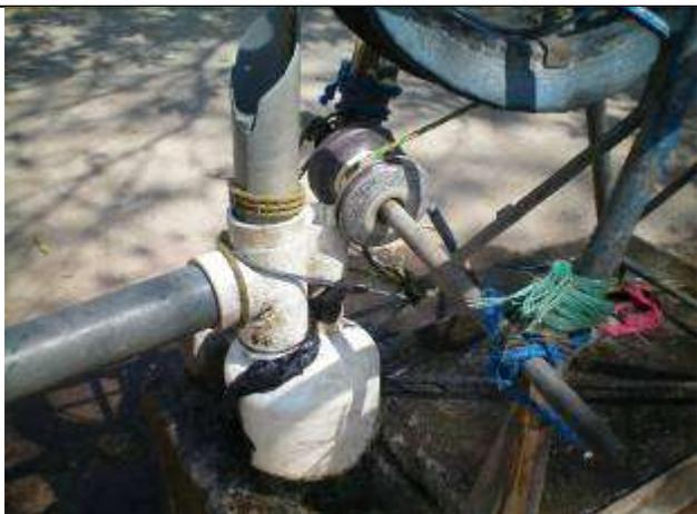
*It is repaired with basic tools and materials like rubber strips but **after 15 years of communal use it still works fine.***
