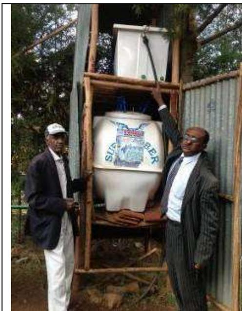
***The top tank is filled up with a hose from the piped water system which is not guaranteed safe to drink. The Filter capacity of this combination is ca 1000 litres per day.***
