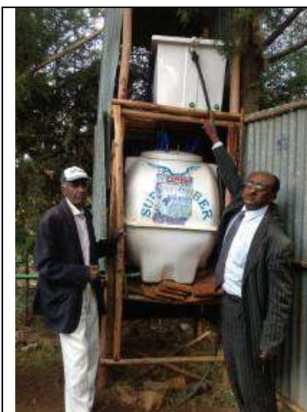
*School in Daleti, Mr Admasu Tesfaye (Righth) showing the feed in pipe through which the unclean water from a well is pumped into the upper feeding tank.*
