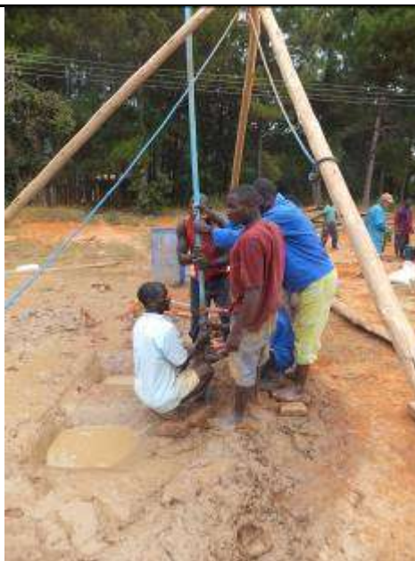
Manual tube well drilling, to 40 m
